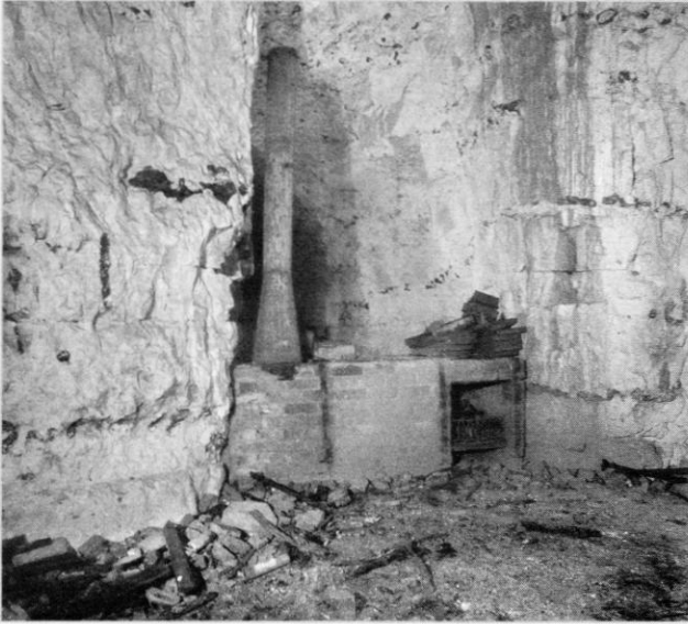
This picture shows the old stove at the bottom of the western shaft. Its chimney used to run up the shaft to the open air. The trays piled on the left of the stove were used to place the small tins of silica gel on, so that they could be placed in the oven. The silica gel was used to keep the documents dry.
